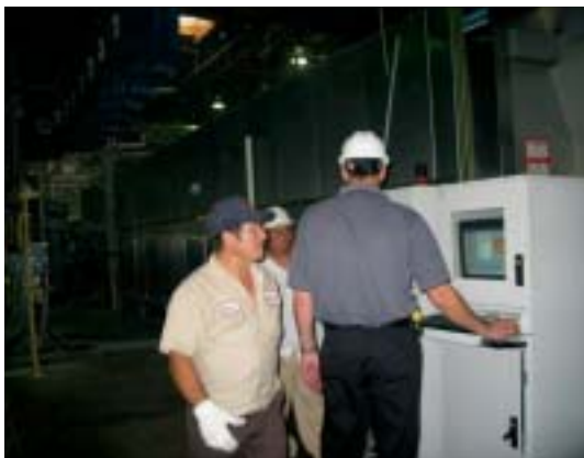
Mission engineers and supervisors check the status of the linen plant's tunnel monitoring system.
